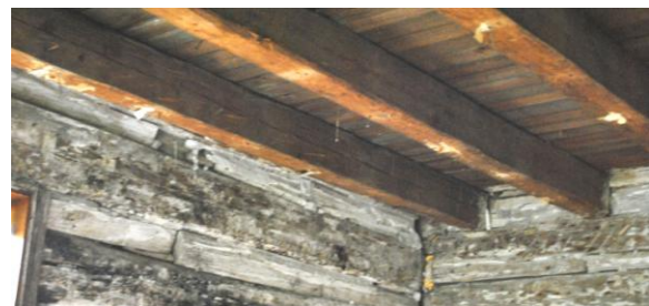
Figure 12 - Second Floor Joists (PSB)
