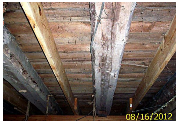
Figure 11 - First Floor Log Joists
