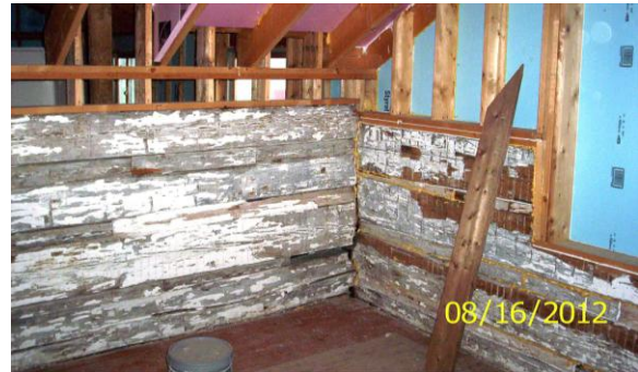
Figure 10 - Second Floor – Briley Log Walls
