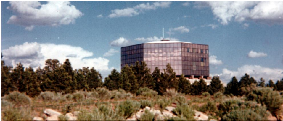
Figure 8 - Main Building of Tsaile' Campus – 6/1991
