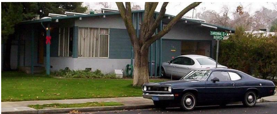
Figure 32 - Solar Panels on roof – 12/2005
