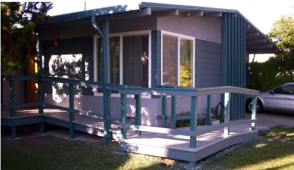
Figure 27 – New Windows and Wheelchair Ramp - 4/2009
