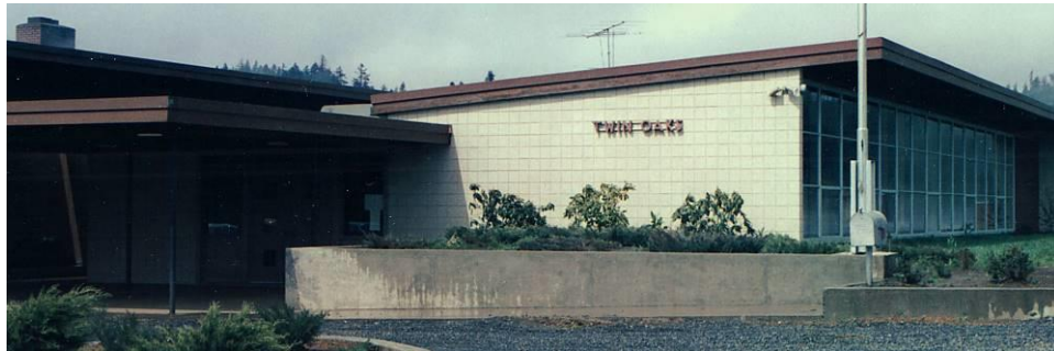
Figure 33 - Twin Oaks Elementary - 1962
