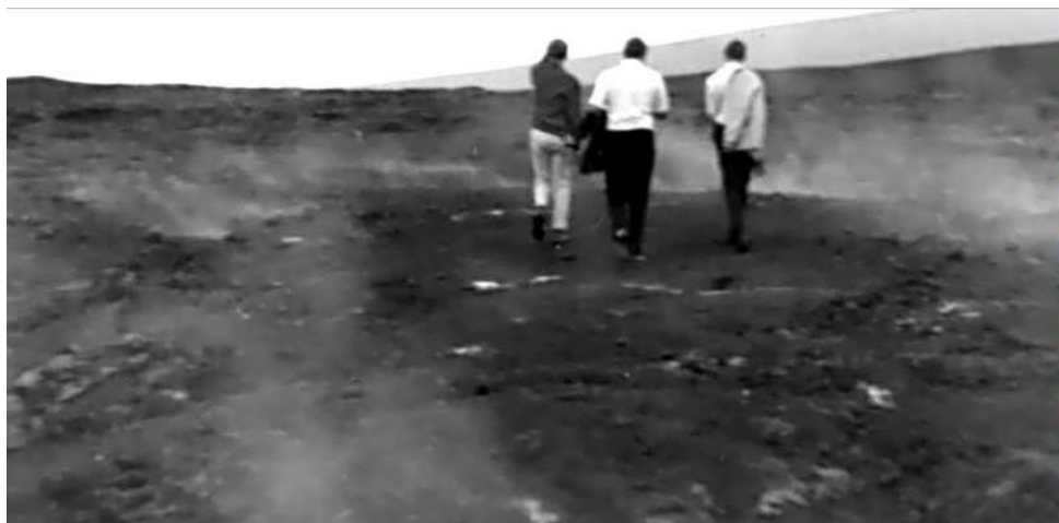
Figure 8 - Pele Trail to Halema’uma’u Fire Pit - 1/1968
