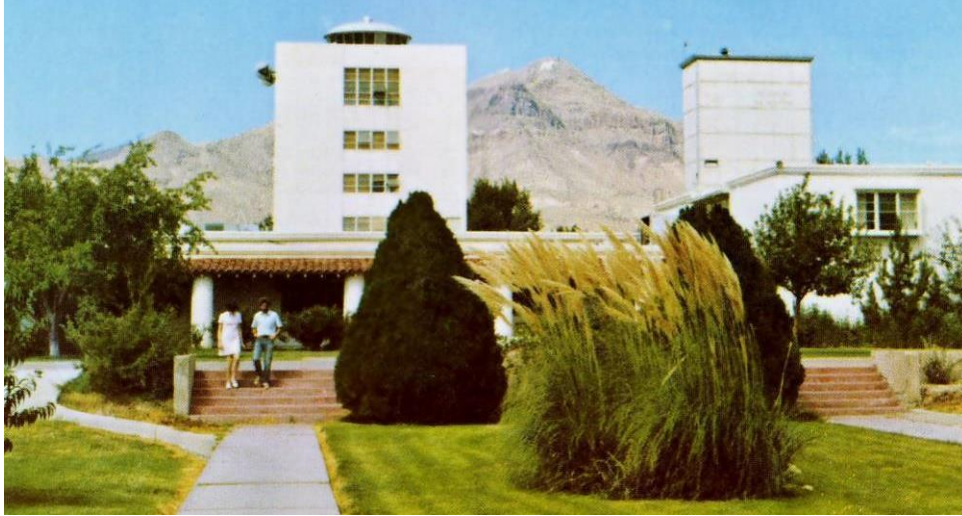
Figure 16 - Workman Computer Center and Bureau of Mines (NMIMT 1975) Kimberly (d.2019) and Earl Eiland descend the steps.
