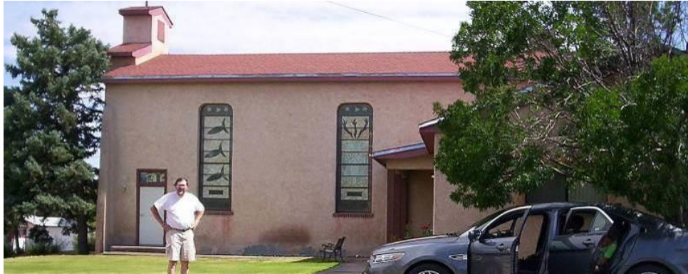
Figure 56 - St. Paul United Methodist Church, Socorro - 2012
