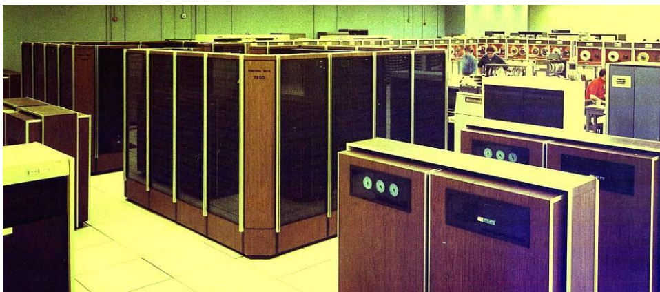
Figure 30 - CDC7600's Computer Room (LLL 1979)
