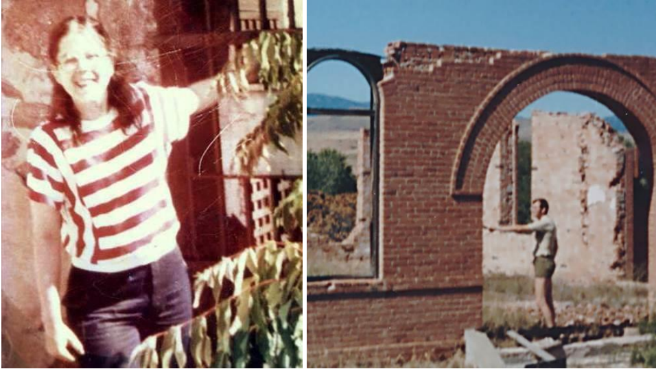
Figure 67 – Dismantled Courthouse, Hillsboro, NM – 10/1982
