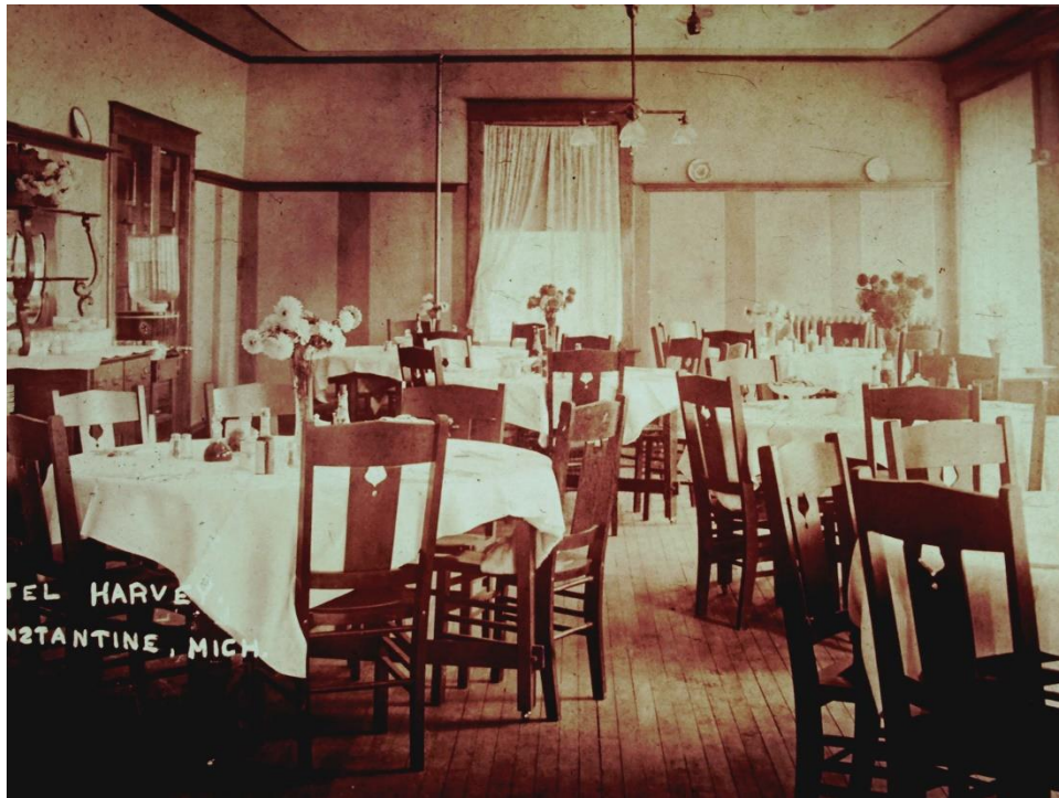
Figure 30 – Hotel Harvey Dining Room – c.1907 (Courtesy of D.Harrison)
