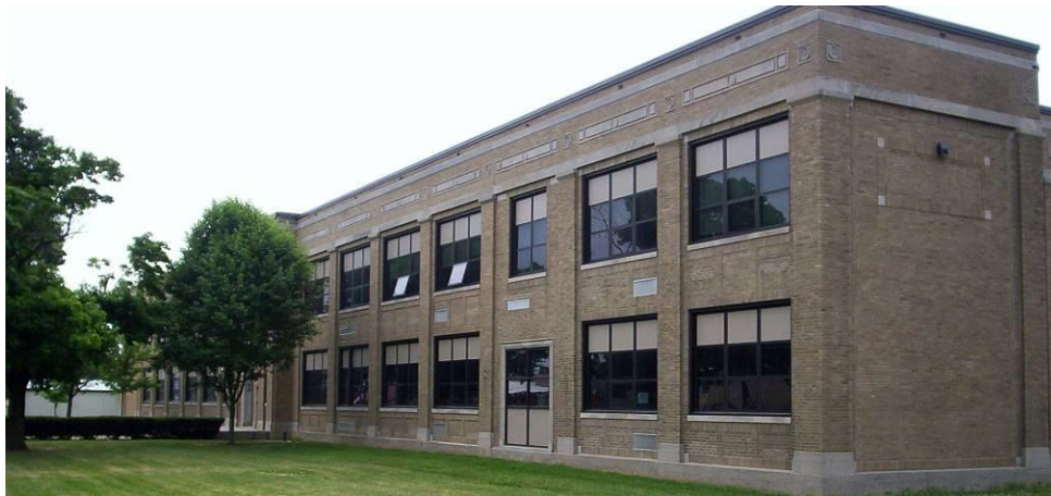
Figure 41 - Adams Elementary rebuilt in 1926 (H. Briley 6/2016)
