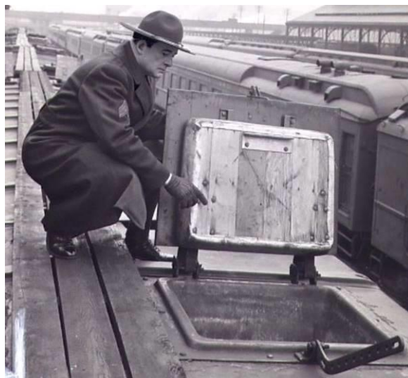
Figure 18 - Refrigerator Car Trap Door - 1940 (Travis Harry)
