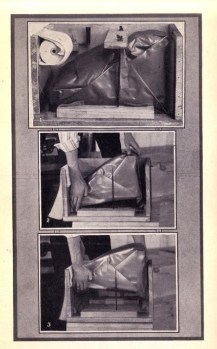
Cut view of SUNDSTRAND packing case showing correct method of unpacking.
